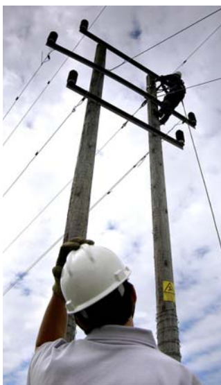
Cable management in action
